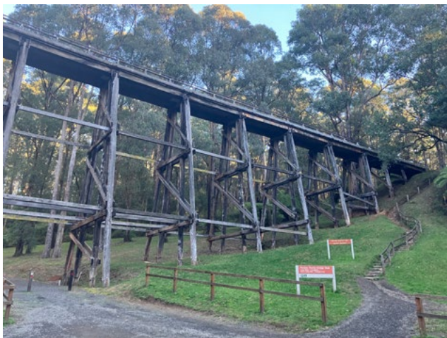
Photo 13 – Noojee trestle bridge (credit: DEECA)
