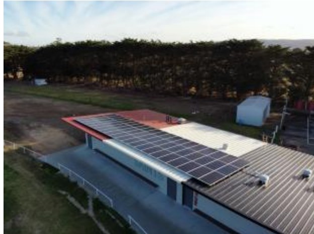
1 - Cowwarr Rec Reserve 20kw solar installation plus Tesla battery enables savings of $5000 to be used to upgrade facilities
